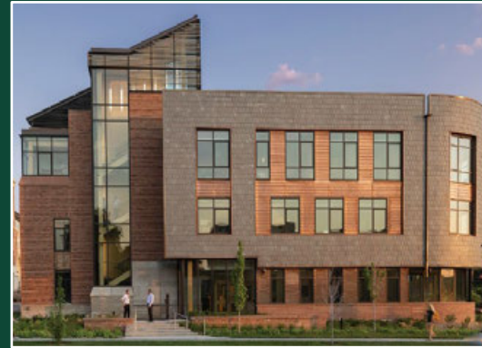
University of Denver Burwell Center for Career Achievement / Lake|Flato Architects / Shears Adkins Rockmore / KL&A Engineers and Builders / Photo © Frank Ooms
