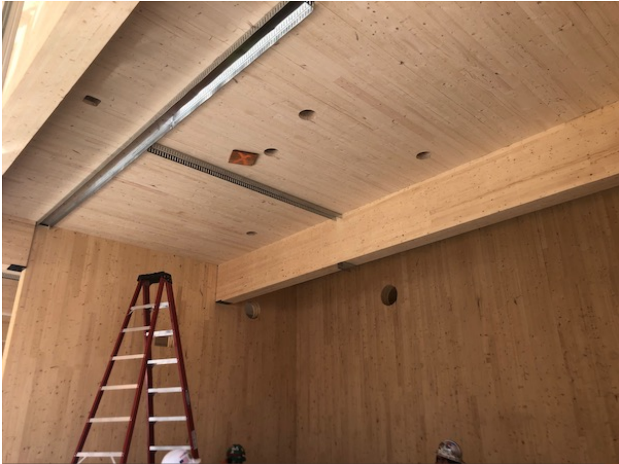
Example of holes in CLT floor panel that do not require reinforcing
