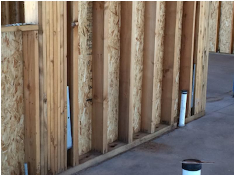
When designing shear wall end posts where holdown anchors are installed, it is common to use posts made from multiple plies of 2x studs (e.g., four 2x6 studs to create one 5.5x6-in post). Section 15.3 of the American Wood Council's (AWC's) National Design Specification<sup>®</sup> (NDS<sup>®</sup>) for Wood Construction includes provisions for built-up columns. However, designers often ask whether these provisions apply to a built-up group of studs
