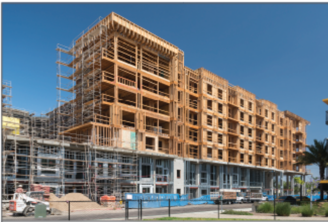
5-over-2 podium building under construction
