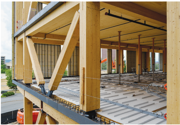
The lateral-resisting system incorporates CLT shear walls and glulam brace frames.
