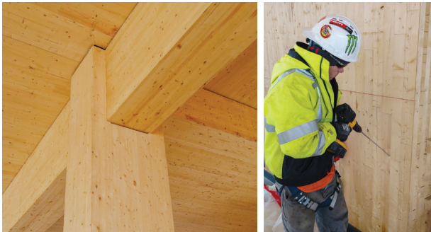
Typical connections included self-tapping wood screws and concealed beam hangers.
