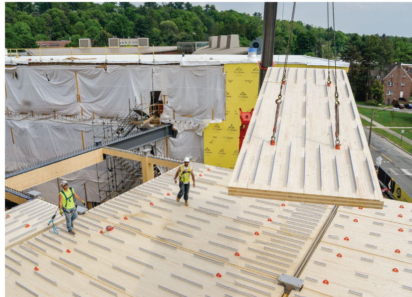
Advantages of mass timber construction include fast installation and a relatively quiet and waste-free job site.
