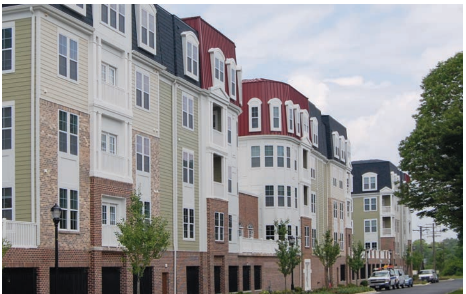
To make The Quarter compatible with the neighborhood architecture, the fourth floor was designed to give the illusion of a three-story building with mansard roofs and attic windows.
