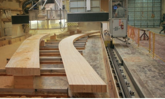
Structurlam Products used a five-axis CNC machine to arch and bevel the huge glulam beams.
