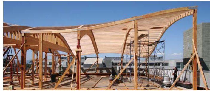
Each CNC-fabricated rafter was custom cut and notched for its specific location in the roof structure. No two were alike.
