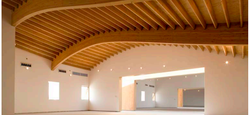
Eric Owen Moss Architects used a sidewall application for lighting and sprinklers to keep the wood roof/ceiling uncluttered.
